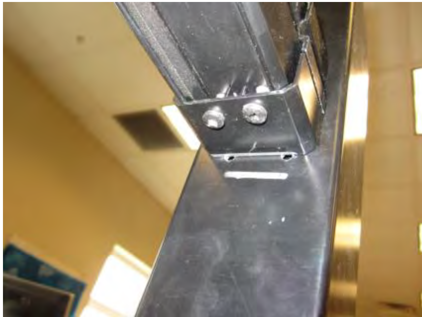
Photo No. 6 Top Rail Bracket-to-Rail Connection
