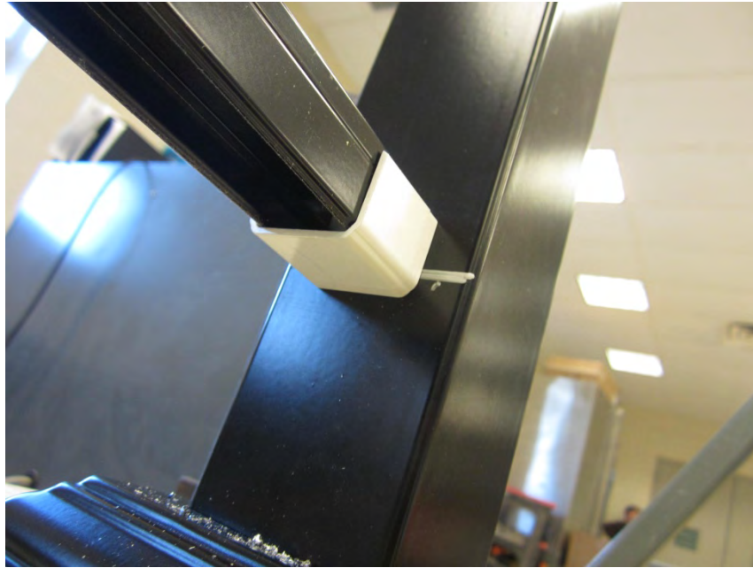
Photo No. 7 Installed Bottom Rail Bracket
