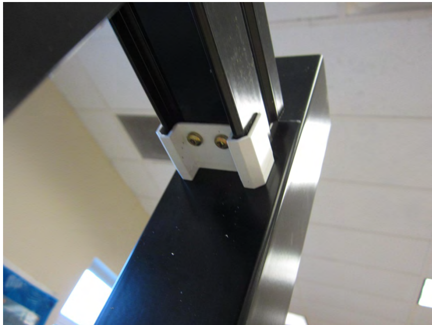
Photo No. 6 Installed Top Rail Bracket
