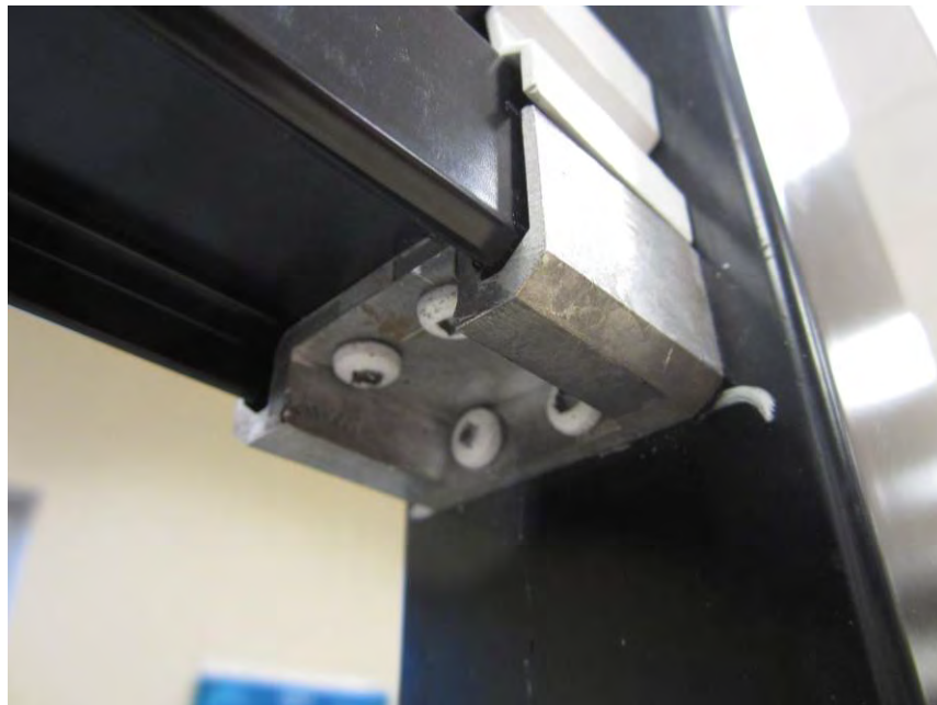
Photo No. 8 Bracket Connection for Top Rail
