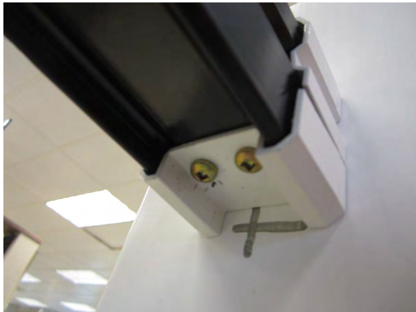
Photo No. 6 Top Rail-Bracket-Post Attachment
