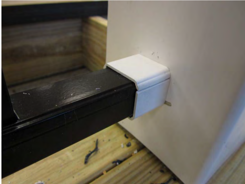
Photo No. 7 Bottom Rail-Bracket-Post Attachment
